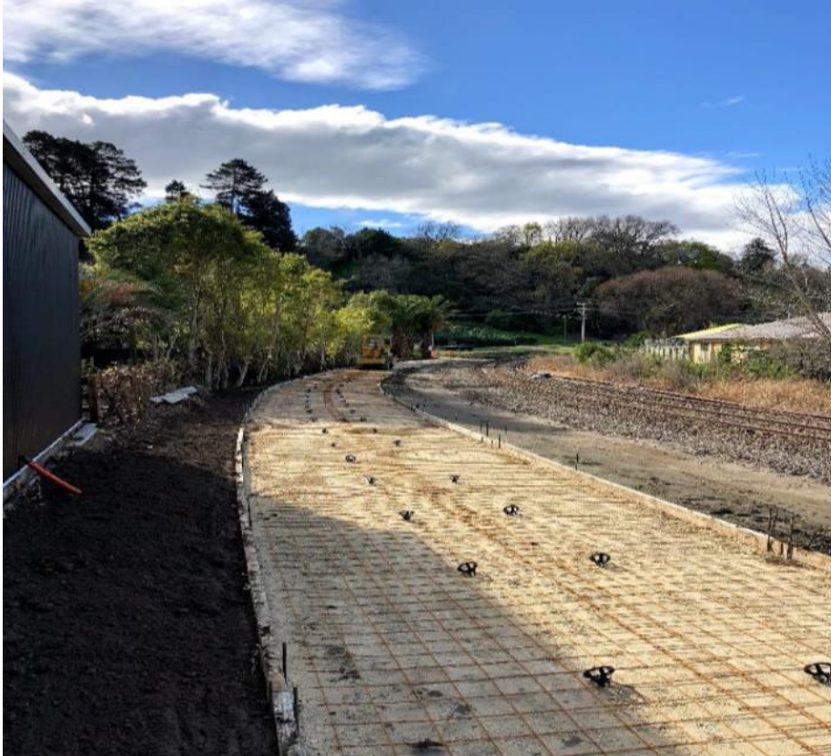
Photo: Preparation of new Te Tuaiwi shared pathway located in Kiwirail corridor between Glasgow Street and SH3, in readiness for concrete
